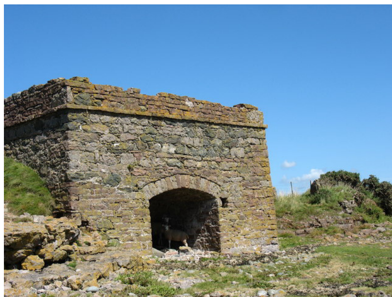
Old Welsh lime kiln (53°08'50.3"N 4°19'39.9"W). "The burning fiery furnace of Dan. 3:6, etc., must have been similar to our common lime-kiln, with a perpendicular shaft from the top and an opening at the bottom for extracting the fused lime..." — Montgomery, A Critical and Exegetical Commentary on the Book of Daniel , 202. Image courtesy of Eric Jones , 2007. This image is licensed under a Creative Commons Attribution-Share Alike 2.0 license .
